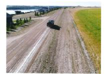
applied to South Memorial Drive and will be completed by August 28<sup>th</sup>. The product is used for new roads to bind the clay content resulting in long term surface retention and considerably reduced maintenance. The application of this durable product will eliminate the annual application of normal dust control product at a fraction of the cost. The results of the treatment will be evaluated as we move forward with our access road development.
